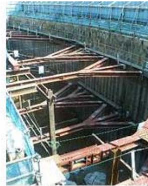
Earth Retaining wall measurement site
