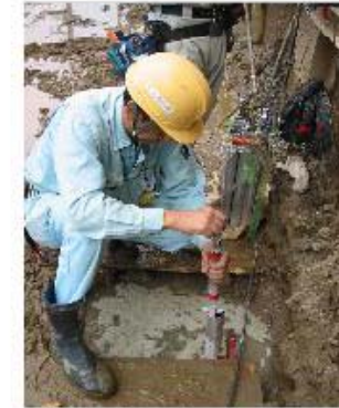
Installation of a multi-layer Clinometer
